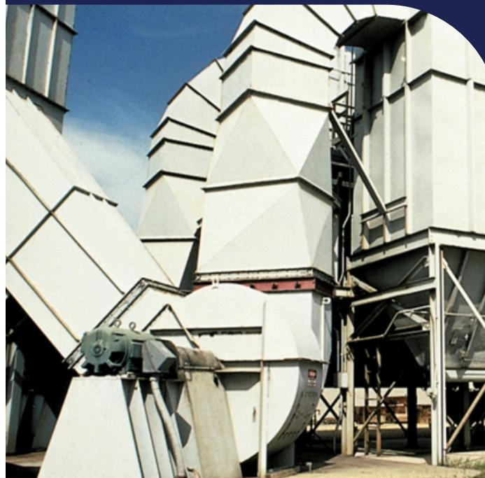
Designed to handle high-volume dust loads, a dust collector system consists of a blower, dust filter, a filter-cleaning system, and a dust receptacle or dust removal system.
